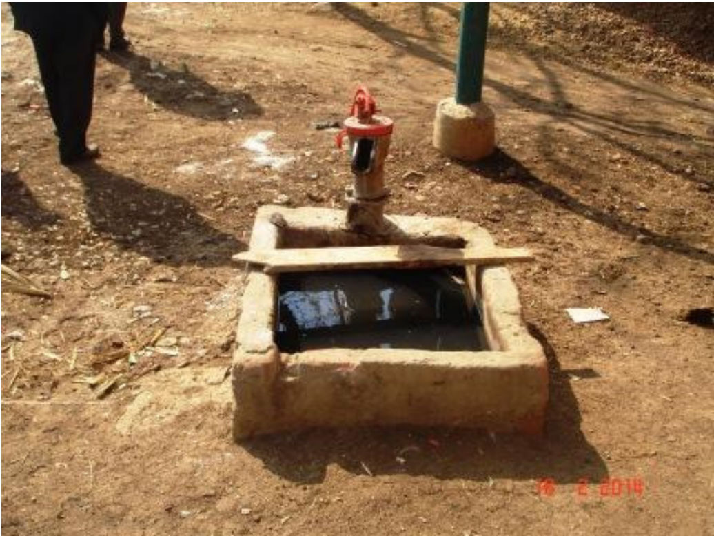
At the beginning the habitants used this primitive bump to get their drinking water. Actually they get waste water at depth 10 to 12 meters .This pump will be go away
